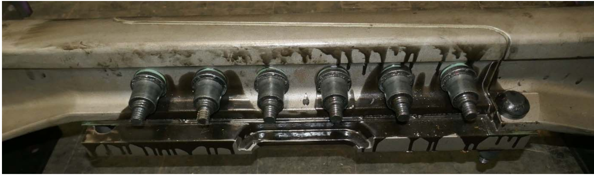
Figure 1: View of insulated joint "ABJ"
